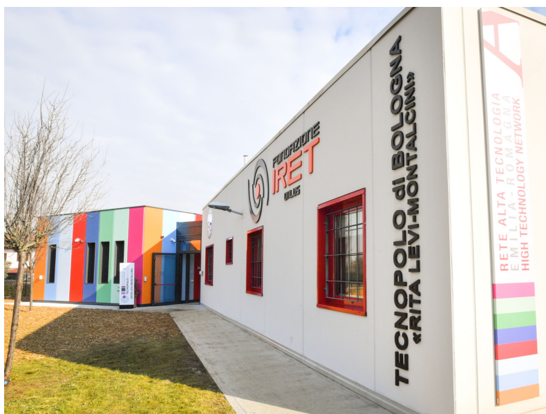
Fig. 1: IRET Foundation, managing body of the Bologna-Ozzano "Rita Levi-Montalcini" Technopole
