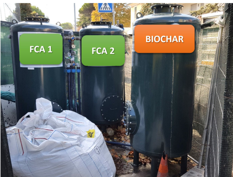
Fig. 3: Application of biochar for water remediation in a Pump & Treat plant
